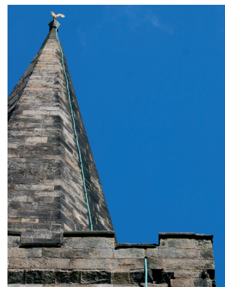
Lightning conductor, St Alkmund's
